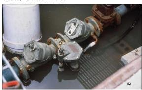
Common Hazard: Incorrectly Installed Backflow Preventers
